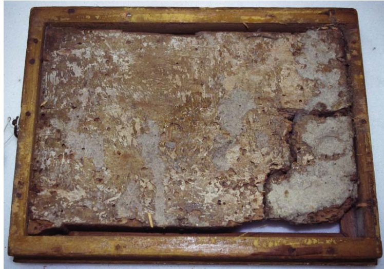
Figure 8 Virgin and Child Eleousa, reverse showing previous repairs to original panel
